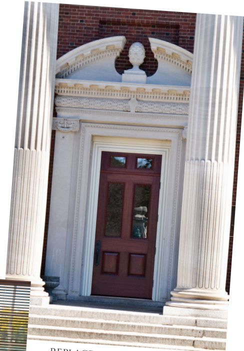
REPLACEMENT OF HENNESSY HALL FRONT DOORS, 2008-2009
